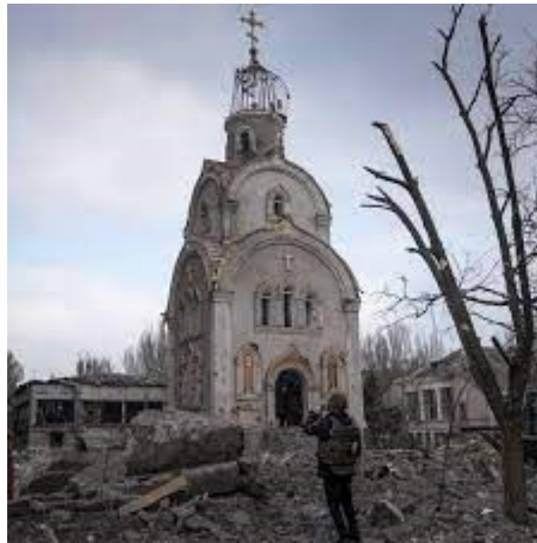
Damaged church in Mariupol, Ukraine. -The Guardian
