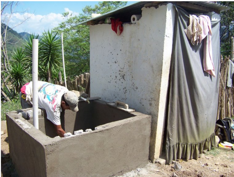
Building a pila (water cistern) in Honduras 2008
